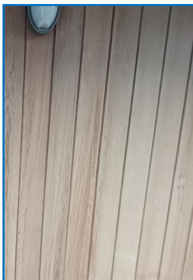
Figure 10: Wall Type 1 Vertical Cedar Wood Cladding
