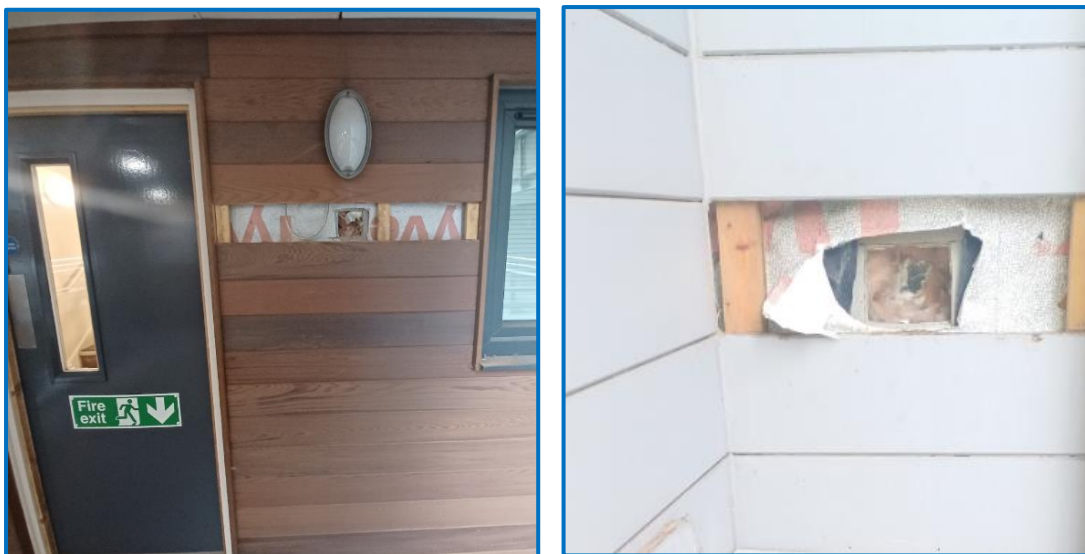
Figure 12: Wall Type 3 – Horizontal Cedar Wood Cladding
