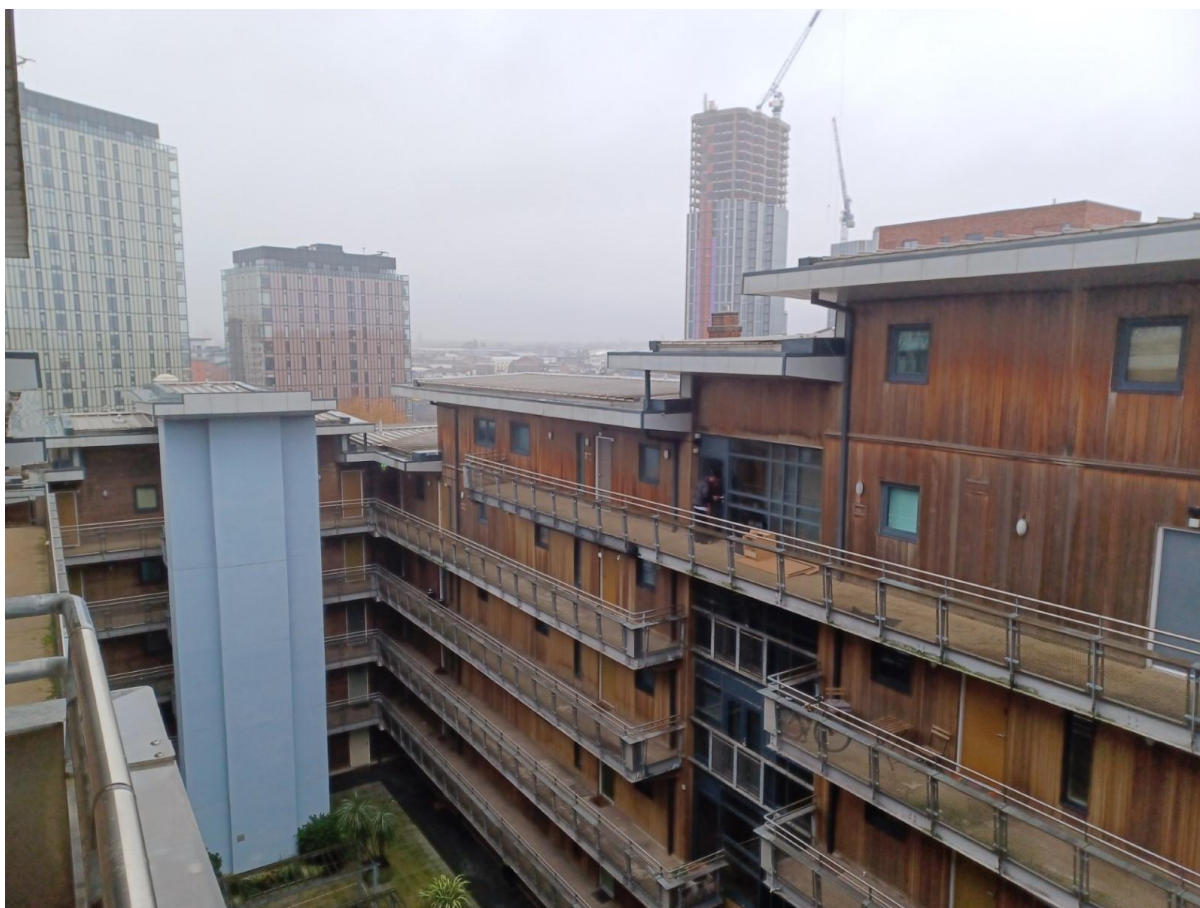
Figure 3 Balcony approaches single means of escape
