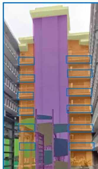
Figure 7 Simpson Street elevation extent of cladding
