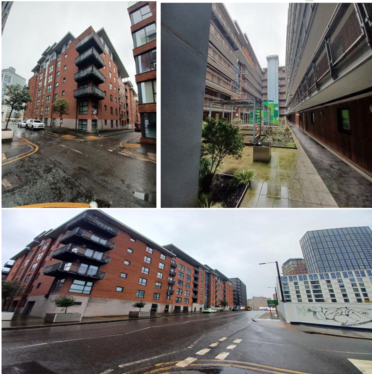
Figure 10 The Linx Building
