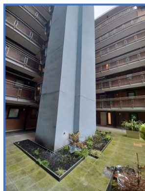
Figure 12: Wall Type 6 – Insulated Render
