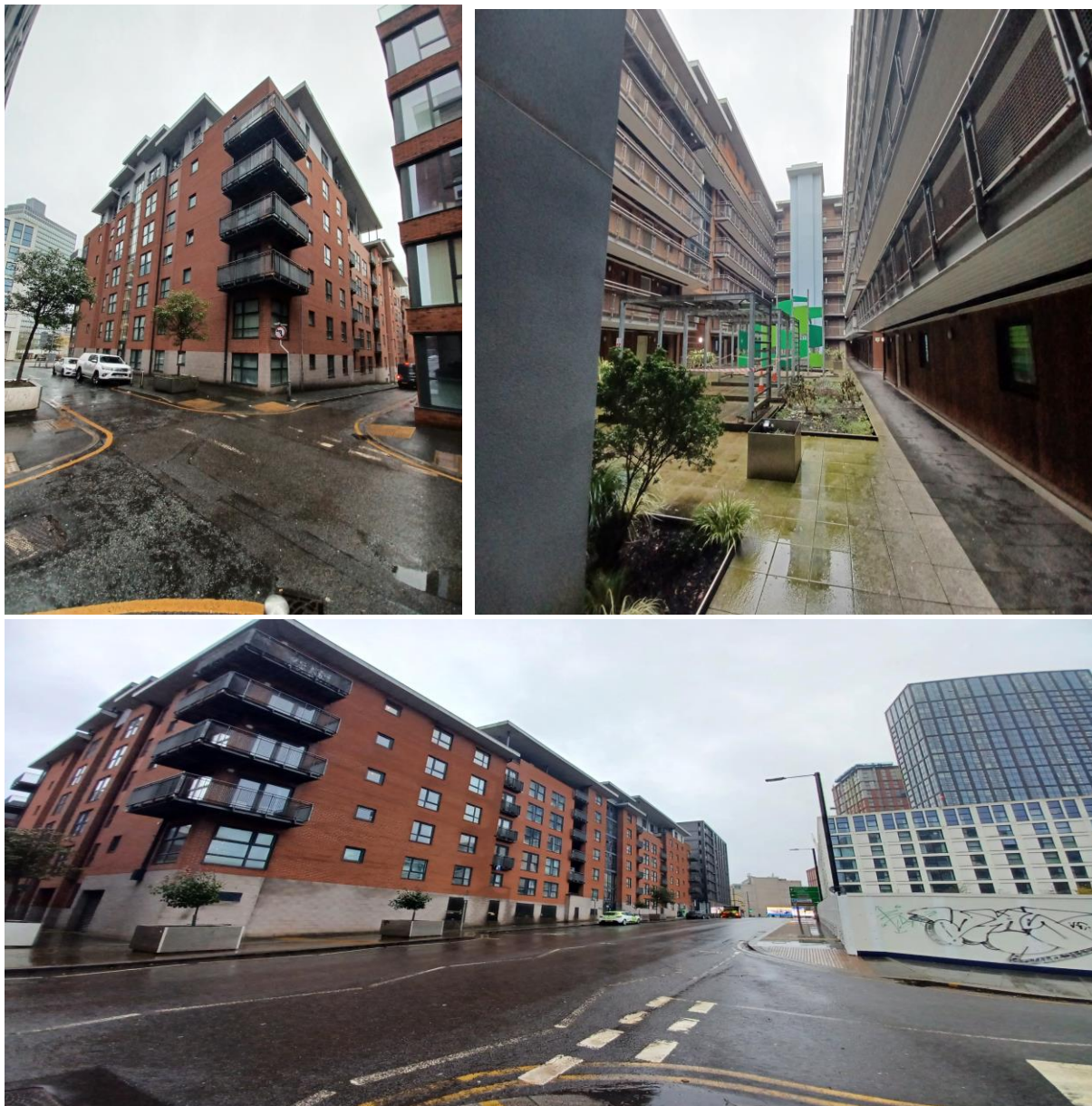
Figure 1 The Linx Building
