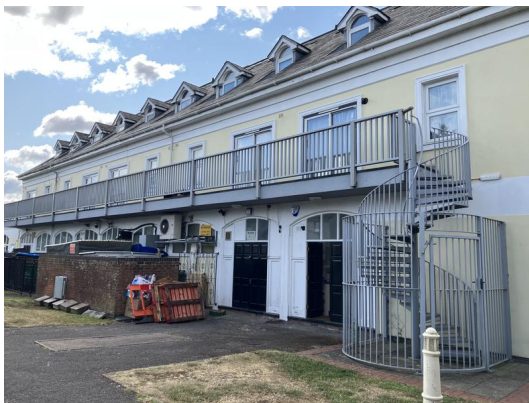
Photo 24 - Secondary escape to apartments 22-30
