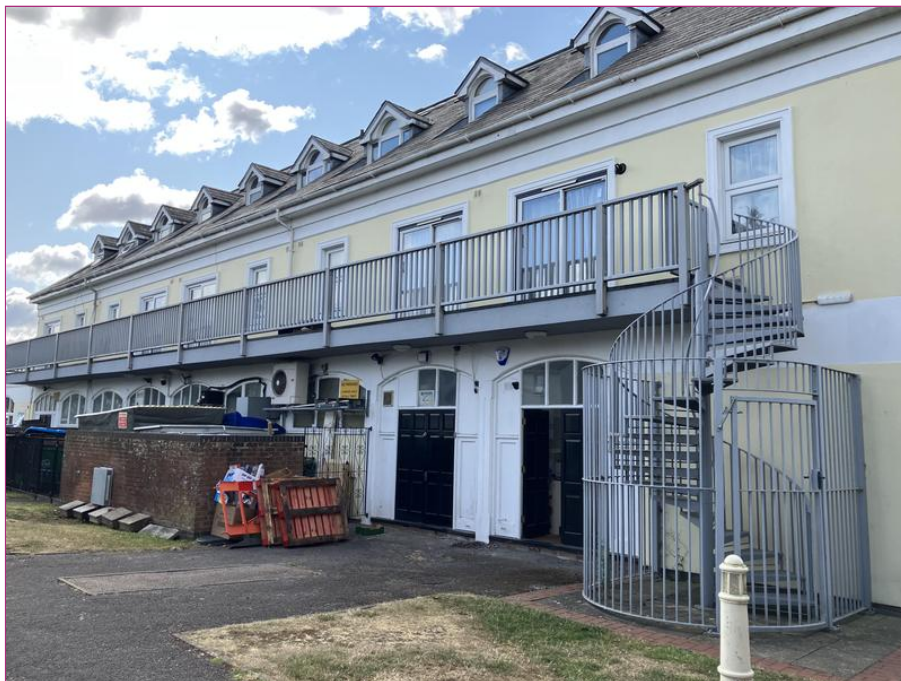
Photo 24 - Secondary escape to apartments 22-30
